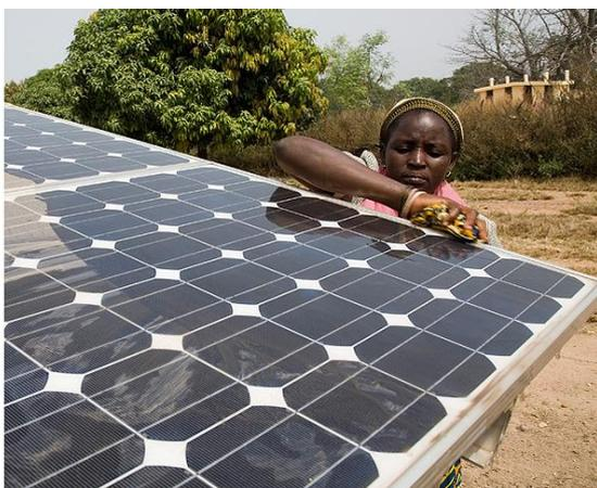
**Figure 5: A woman cleans a solar panel that powers the drip irrigation system in Benin**
