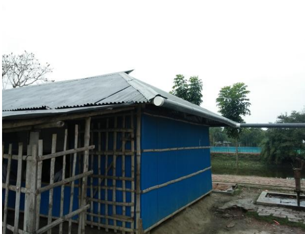
Photo 15: Rainwater collection using pipes and rooftop in Darunmallik of Paikgachha, Khulna
