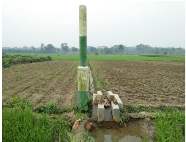
Photo 2: Supply line of Solar Irrigation Pump (SIP) in Doyapur of Kaliganj, Jhenaidah
