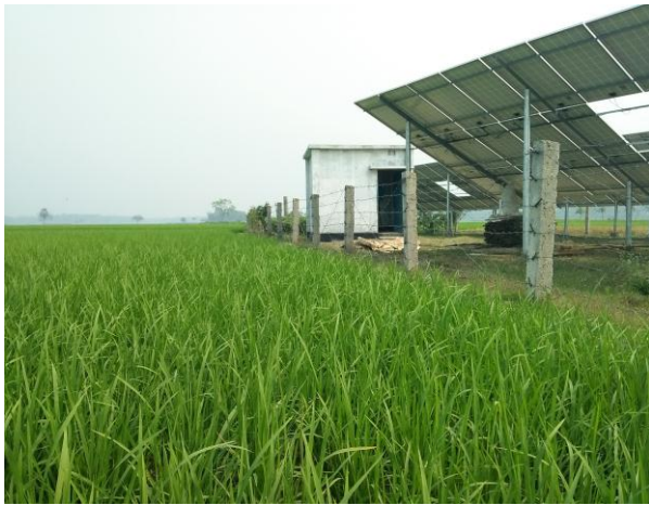
Photo 3: Solar Irrigation Pump (SIP) in Jagannathpur of Kaliganj, Jhenaidah
