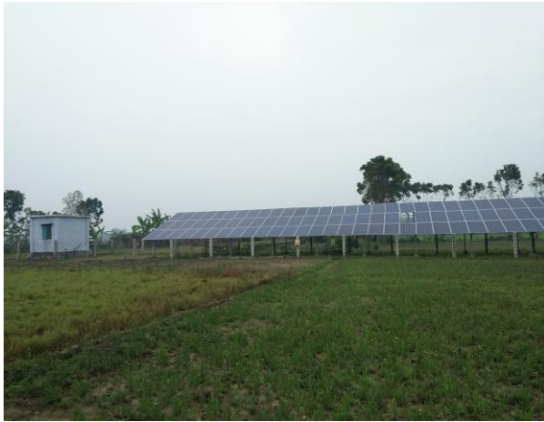
Photo 1: Solar Irrigation Pump (SIP) in Doyapur of Kaliganj, Jhenaidah
