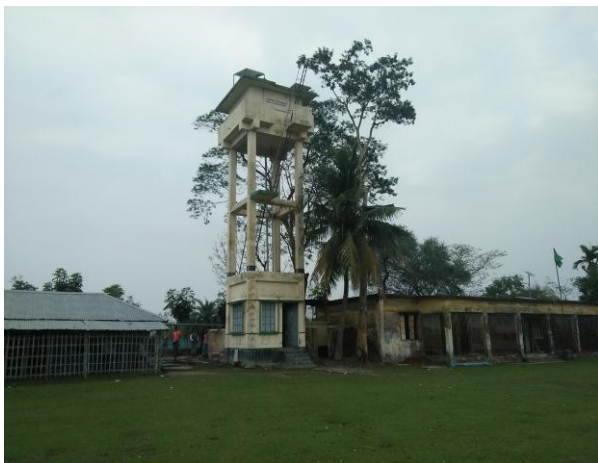
Photo 11: Solar Based Drinking Water Supply (Solar DWS) in Darunmallik of Paikgachha, Khulna
