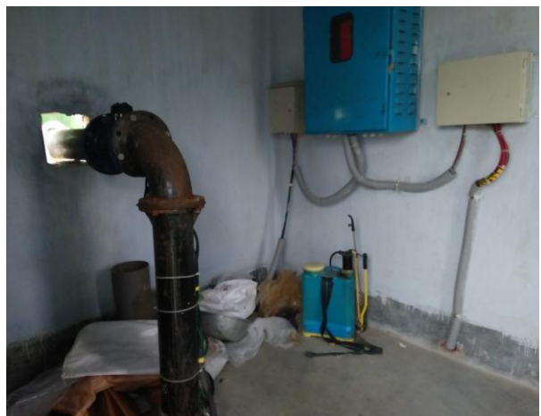
Photo 6: Inside of the controller, motor and connector panel housing in Doyapur of Kaliganj, Jhenaidah
