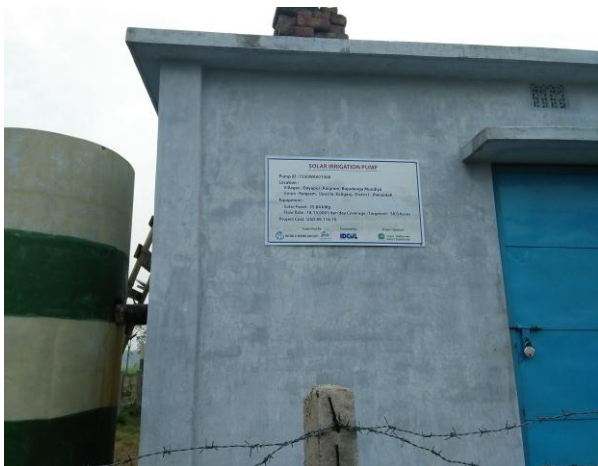
Photo 5: Solar Irrigation Pump (SIP) controller, motor and connector panel housing in Doyapur of Kaliganj, Jhenaidah
