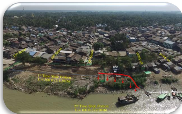
Nyaung Done Town river bank protection works
