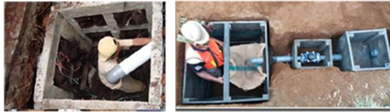
Model of infiltration wells and recharge wells from rooftop rainwater harvesting planned on site (Rohman, 2020)
