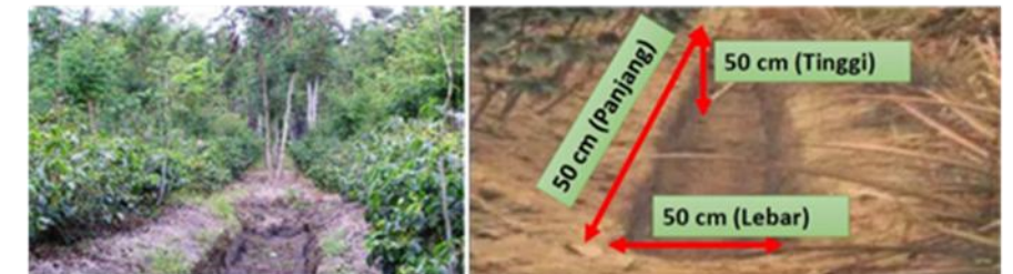
Model of infiltration trench planned on site in Indonesia language where shows the dimension of long (panjang), wide (lebar) and depth (tinggi) (Rohman, 2020)
