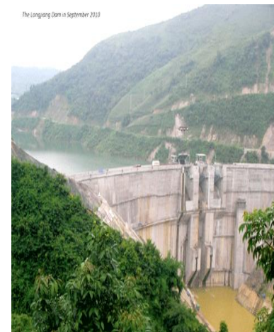
LONGYANG CONCRETE ARCH DAM ON SHWELI RIVER AT CHINA SIDE ABOUT 25 km NORTH OF MYANMAR-CHINA BORDER
