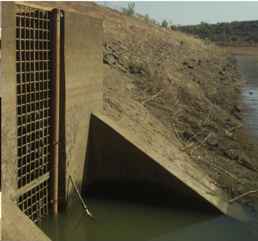
3 water level stations in the reservoirs
