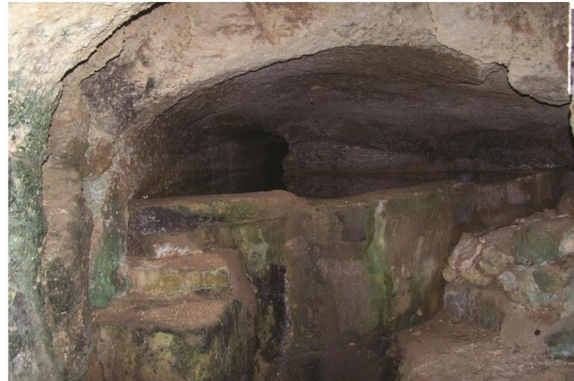
The Lunjzjata perched aquifer gallery and its fronting water reservoir, located in the territory of Rabat, Malta. ©K.Buhagiar
