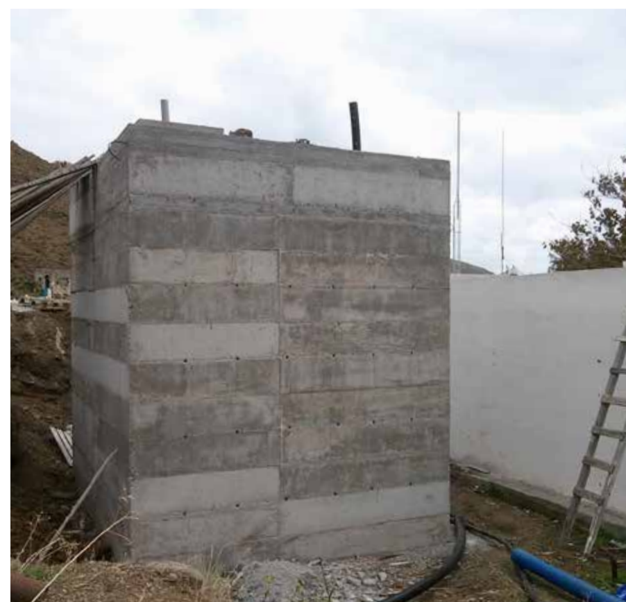
Fig.2: Above: Maintenance of the main municipal water reservoir in Kastello-rizo, Greece (source: GWP-Med) Left: Construction of a concrete reservoir in Astypalea, Greece (source: GWP-Med)
