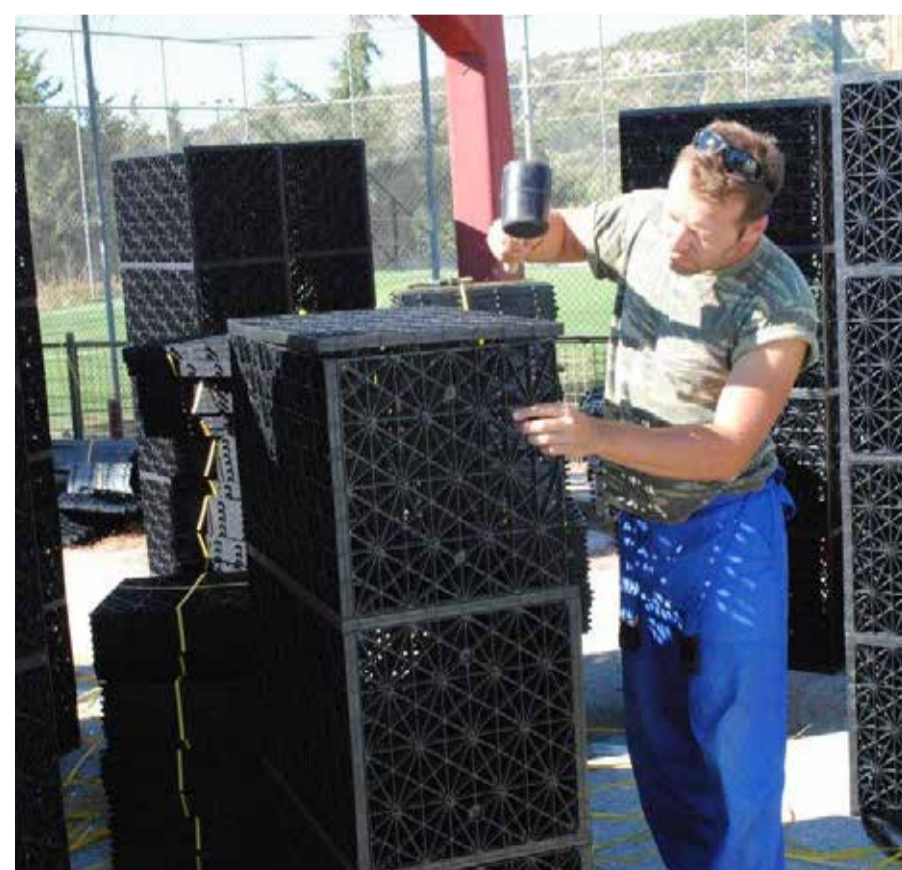
Fig. 7: Above: Installation of a modular tank in Syros Island, Greece. (source: GWP-Med) Left: Modular tank assembling (source: GWP-Med)
