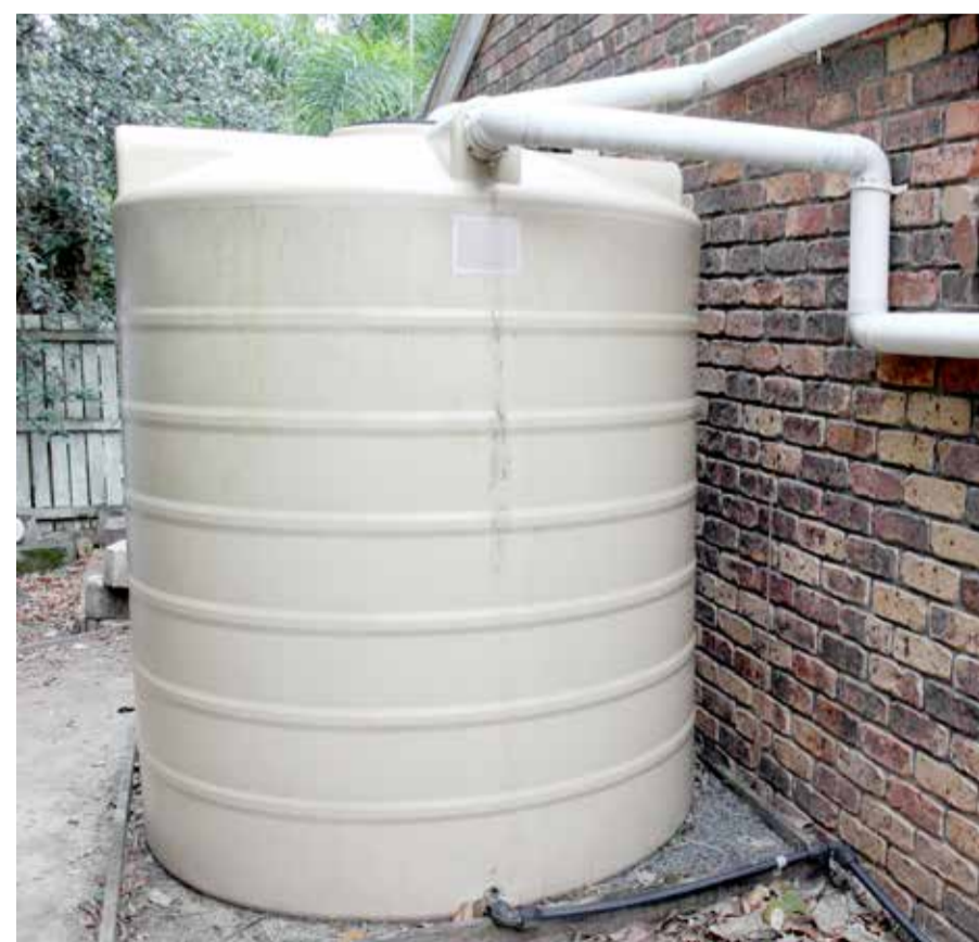
Fig.3: Above: Plastic rainwater harvesting tank installed by UNICEF-Rwanda. (source: E. Dusingizumuremyi, SuSanA Secretariat) Left: Plastic rainwater harvesting tanks (source: Kathie Nichols)
