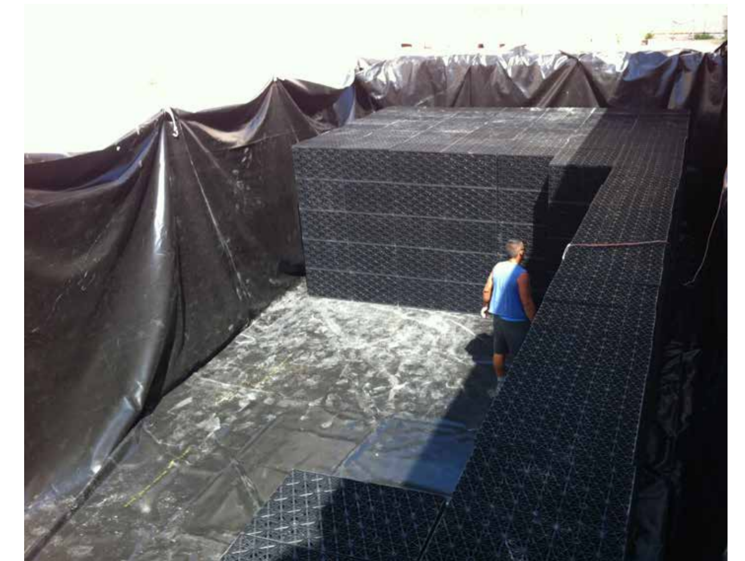
Fig. 8: Installation of a modular tank in Gozo, Malta (source: GWP-Med)
