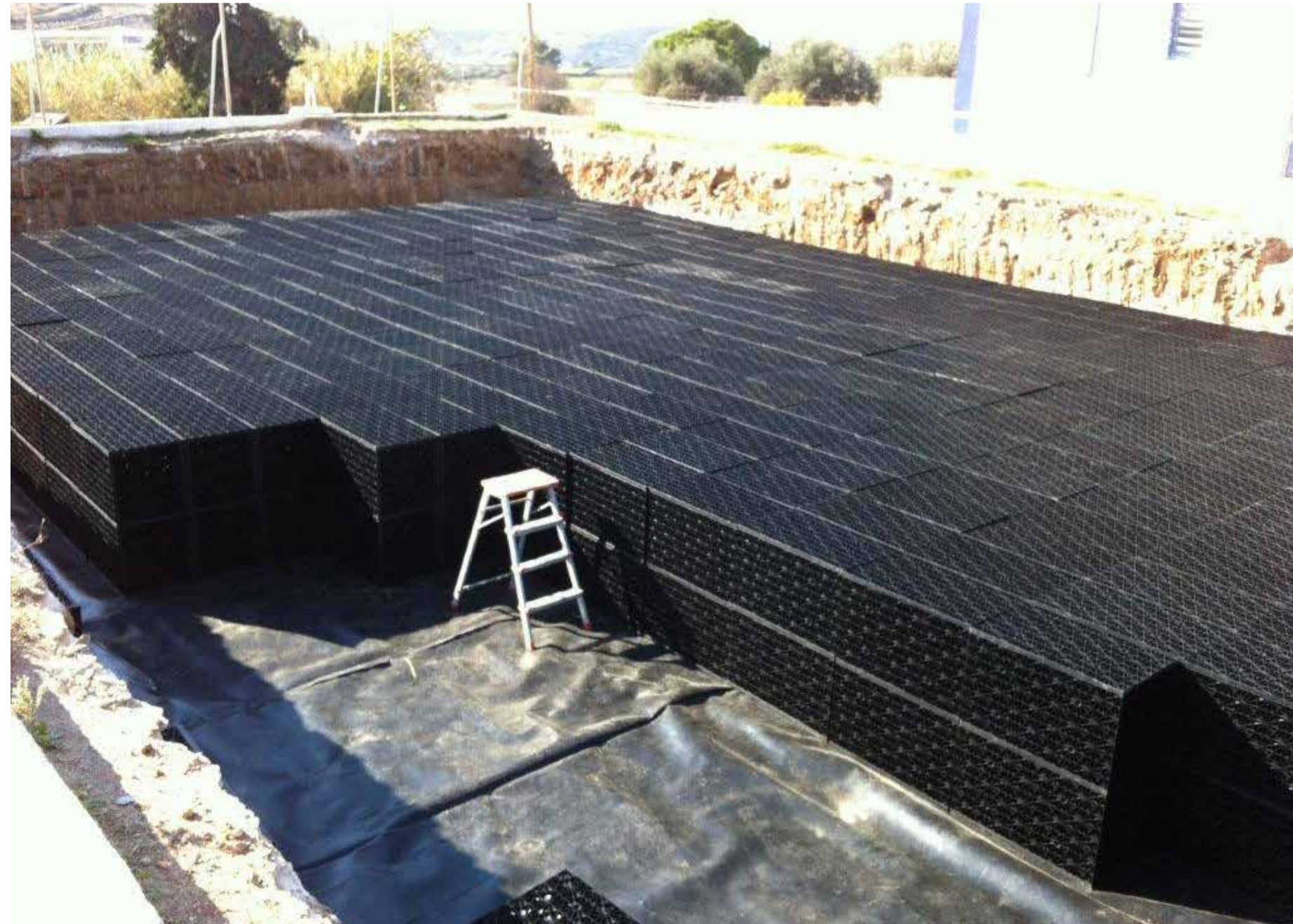
Fig. 7: Above: Installation of a modular tank in Syros Island, Greece. (source: GWP-Med) Left: Modular tank assembling (source: GWP-Med)
