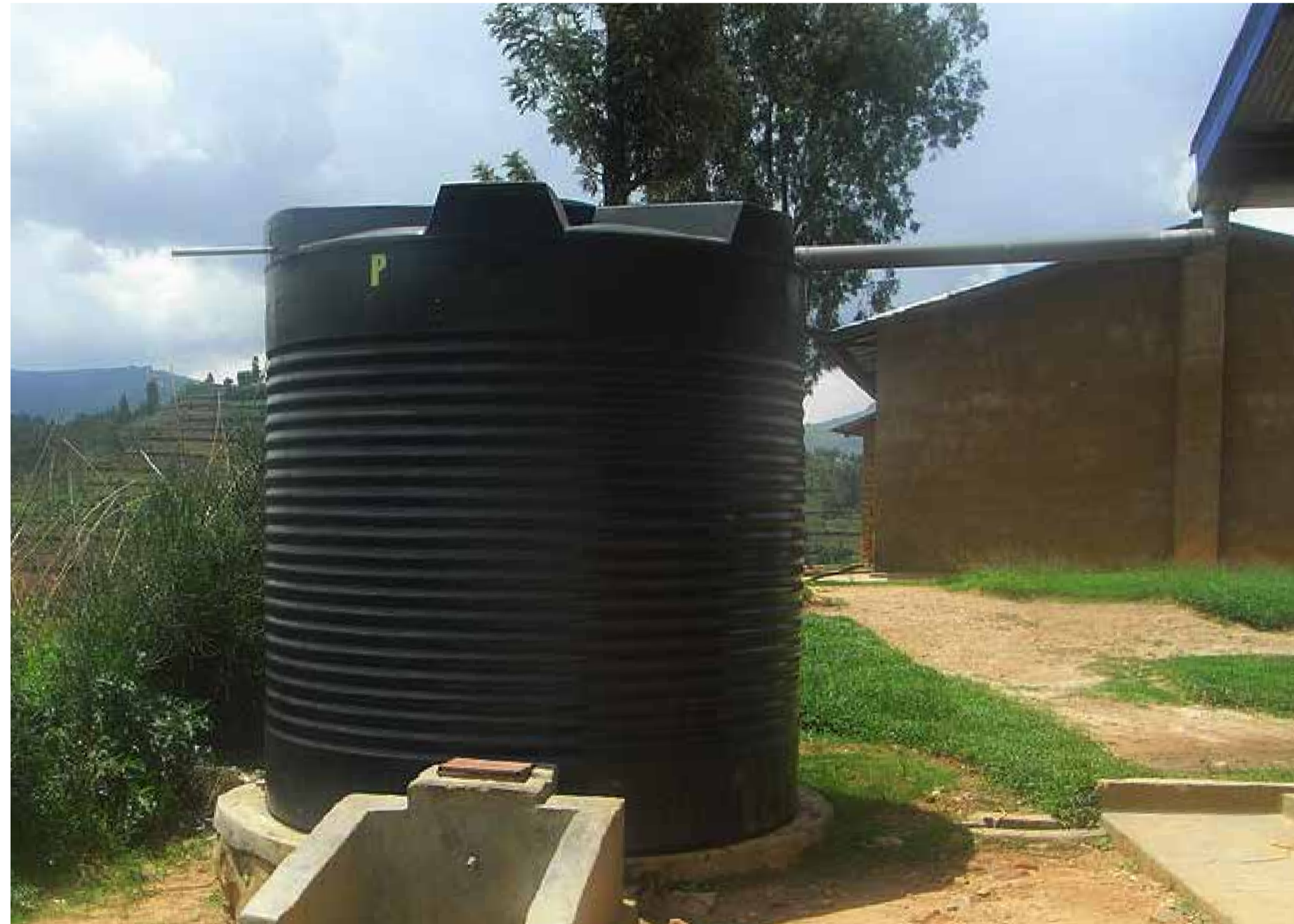
Fig.3: Above: Plastic rainwater harvesting tank installed by UNICEF-Rwanda. (source: E. Dusingizumuremyi, SuSanA Secretariat) Left: Plastic rainwater harvesting tanks (source: Kathie Nichols)
