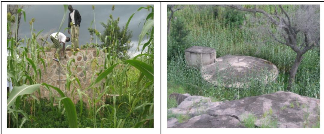
Figure 2: Rock surface water harvesting system with a storage reservoir.
