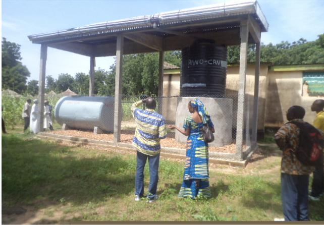
Figure 1: Roof top water harvesting site in meri; one with a metal storage tank and the other with concrete.
