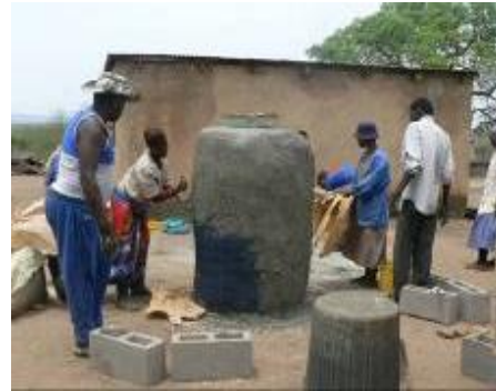
locals constructing a water harvester
