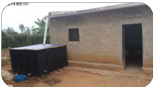
Figure 3: Roof water harvesting to support biogas digestion (Rwanda)
