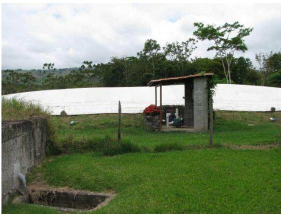
Fig. 2 Biodigestor Produce 498 m<sup>3</sup>
