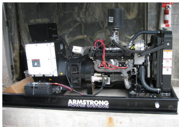
Fig. 3 Biogas-based electricity generation plant
