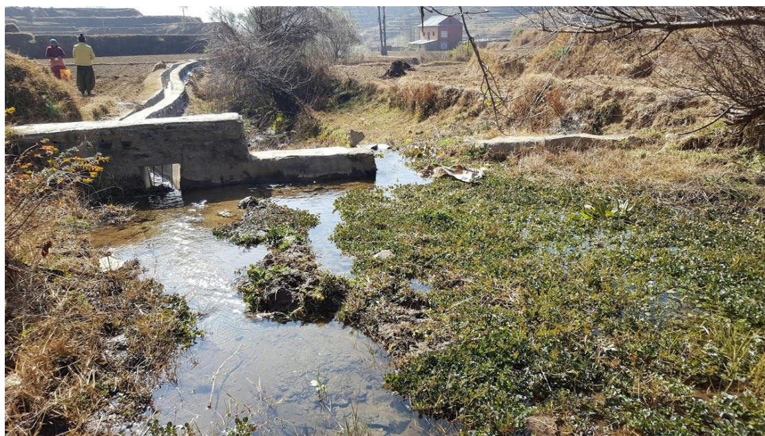
Figure 4 Picture showing a gate system connecting irrigation canals between upstream and downstream farmers in Bajrabarahi (source: NACCFL, 2017)
