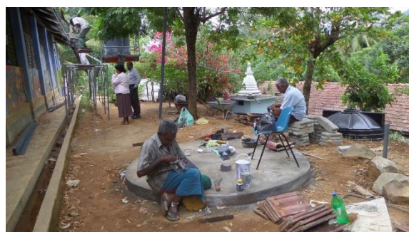
Image 2: Construction of Rainwater Harvesting Systems
