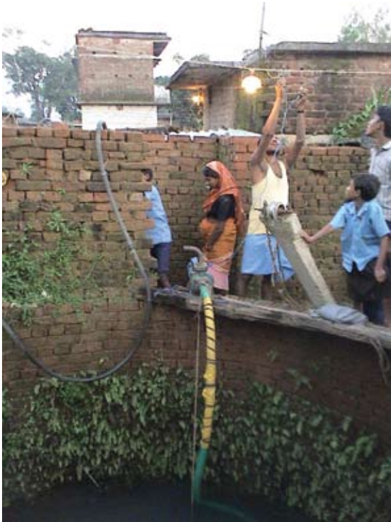
Farmers in Jharkhand State, India tap into local electricity lines to power their pumps.
