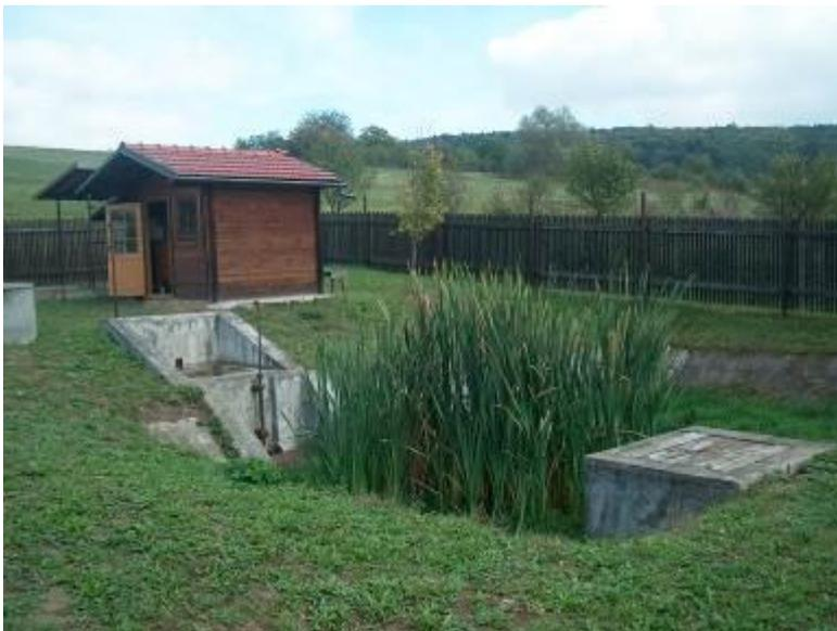
Stormwater retention tank (2006): Well-grown vegetation of *Typha* sp.
