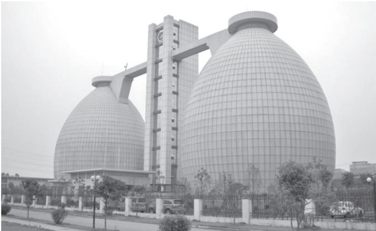
Sludge digester at the Sanjintan wastewater treatment plant in Wuhan, Hubei Province. Source: Arup 2010.
