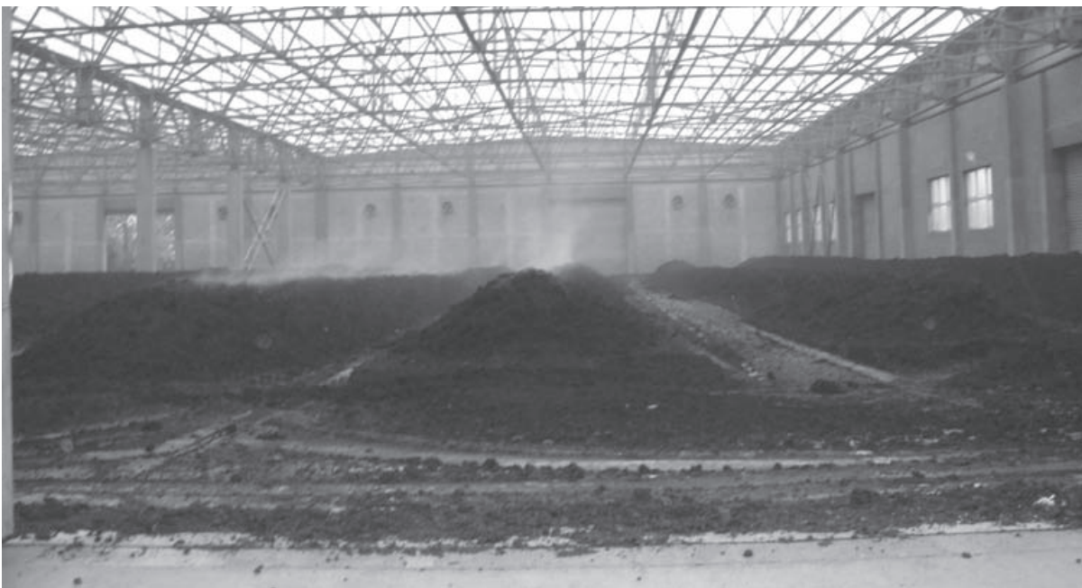
High quality of sludge products must be ensured to overcome resistance to beneficial sludge utilization. Above, the Panggezhuang sludge composting plant in Beijing. Source: AECOM 2010.
