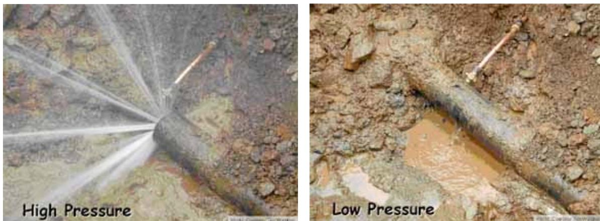
**Figure 7. Burst water main at high and low pressure**
