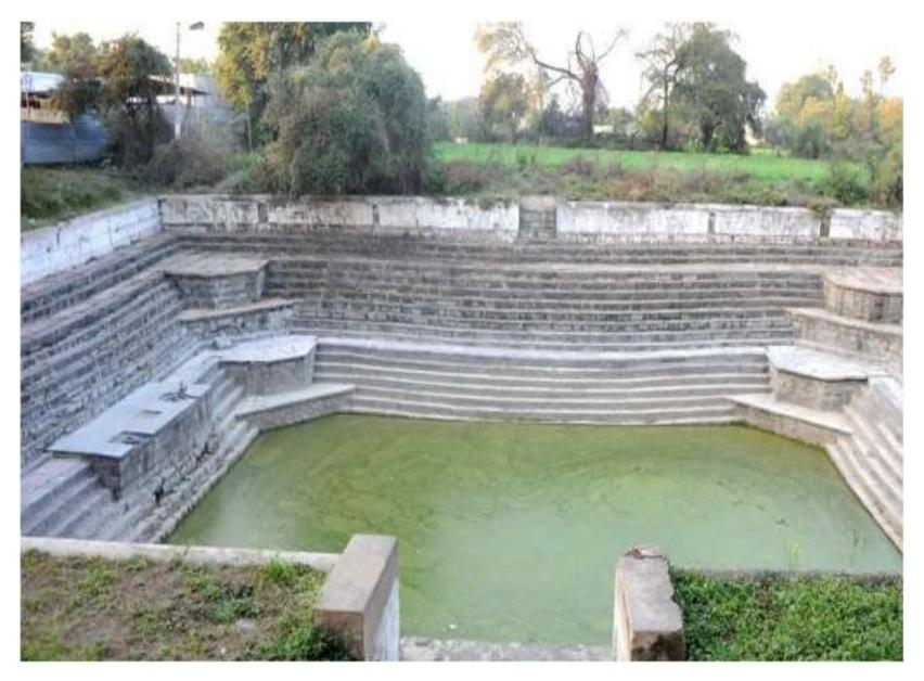
A kund is a saucer-shaped catchment area that gently slope towards the central circular underground well. Its main purpose is to harvest rainwater for drinking. Kunds dot the sandier tracts of western Rajasthan and Gujarat. Traditionally, these well-pits were covered in disinfectant lime and ash, though many modern kunds have been constructed simply with cement. Raja Sur Singh is said to have built the earliest known kunds in the village of Vadi Ka Melan in the year 1607 AD.
