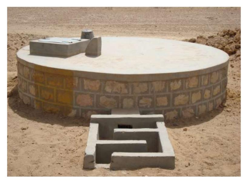
Taanka is a traditional harvesting rainwater technique indigenous to the Thar desert region of Rajasthan. A Taanka is a cylindrical paved underground pit into which rainwater from rooftops, courtyards or artificially prepared catchments flows. An important element of water security in these arid regions, taankas can save families from the everyday drudgery of fetching water from distant sources.
